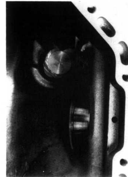
Blanking plug installed
